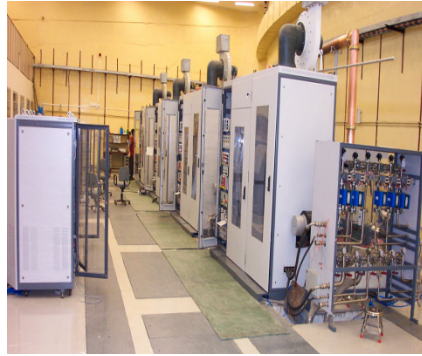
FIGURE 1. High power Klystron based RF amplifiers in Indus-2 SRS
